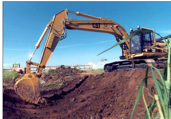
Excavation of ditch soils in Zone 11
