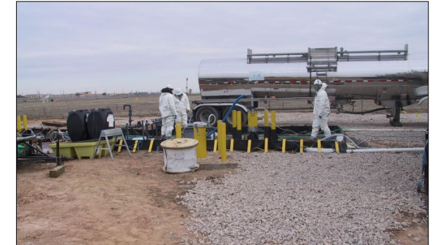
Injecting amendment into perched groundwater to create a permeable treatment zone
