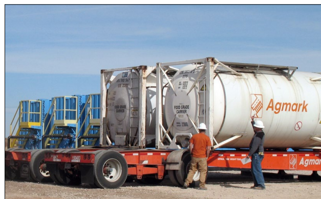
Tankers of food grade soybean oil and lactic acid to be injected into the perched groundwater to create an enhanced anaerobic bioremediation zone
