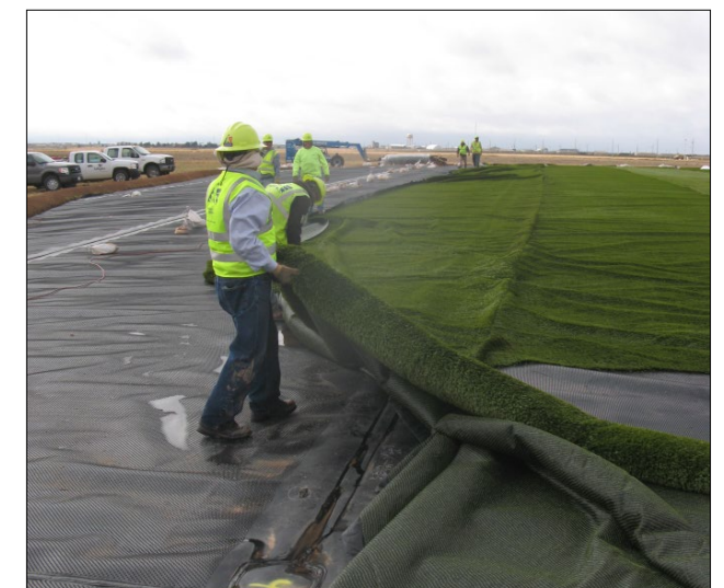
ClosureTurf™ installation
