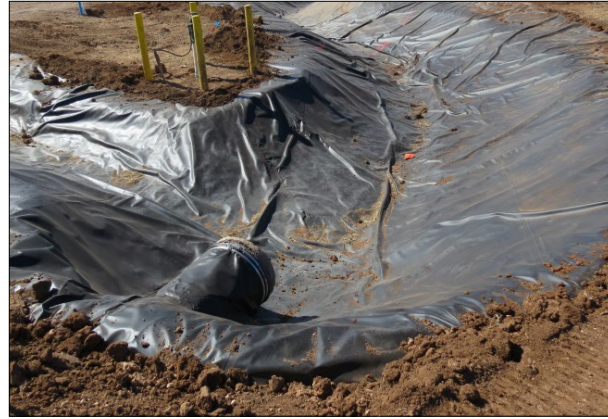
Ditch Liner in Zone 12
