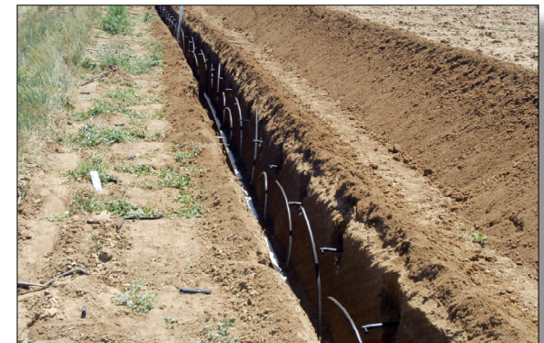
Installation of a subsurface irrigation system near Playa 1.
