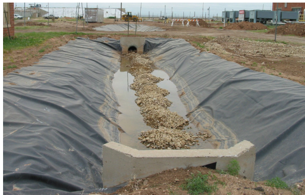
Installation of a ditch liner in Zone 12.
