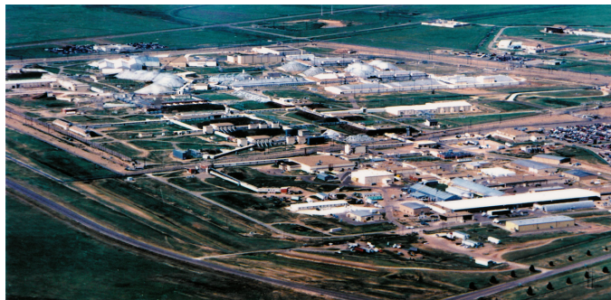
Aerial photograph of Zone 12 at Pantex Plant.
