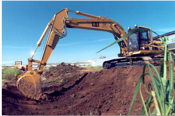
Excavation of ditch soils in Zone 11.
